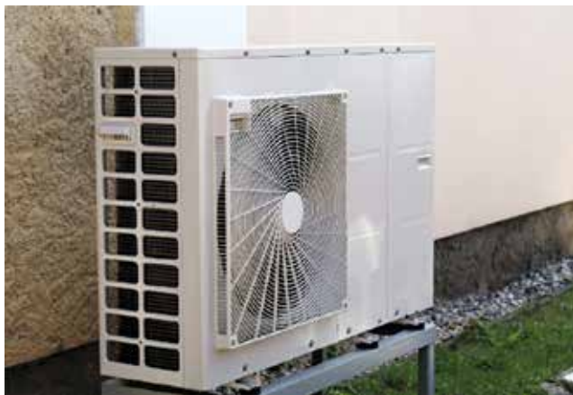
An air-to-water heat pump looks like an air conditioning unit and works like a fridge in reverse.
