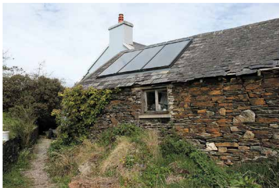
Rooftop solar thermal panels on an outhouse.
